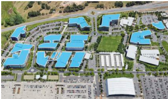
SkySpark implementation which analyses 7500+ data points across a campus of buildings shown in blue
